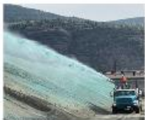
Placing dust suppressant for less active piles
