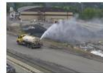
Wetting exposed piles during wind events
