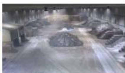
Indoor material handling of Lead concentrate
