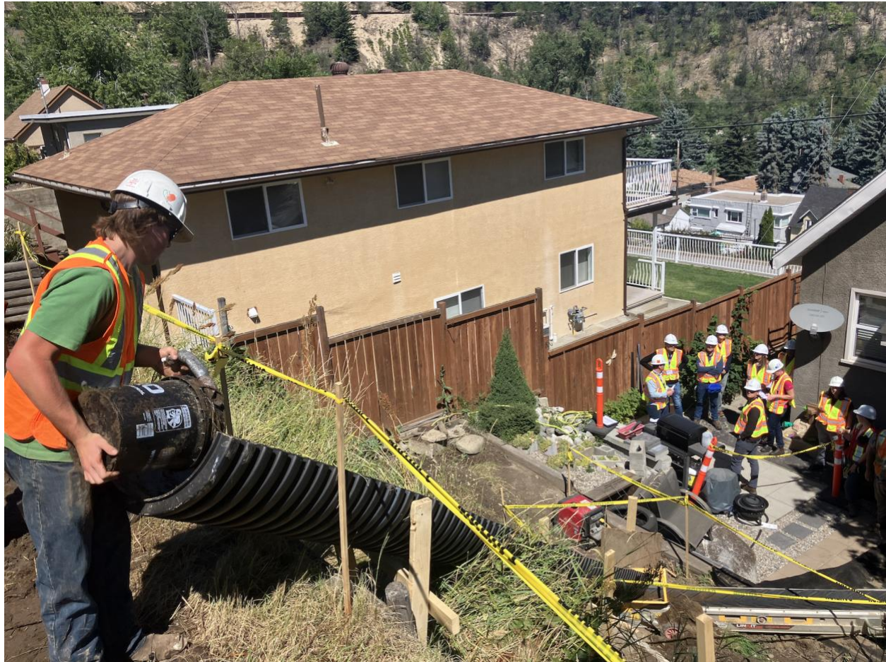
Photo 1: Innovative method used for soil replacement on a tough access property with six steep terraces in Trail.
